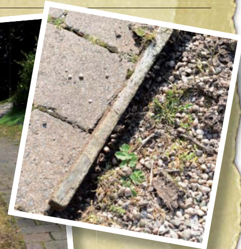
The original rotting timber edging
